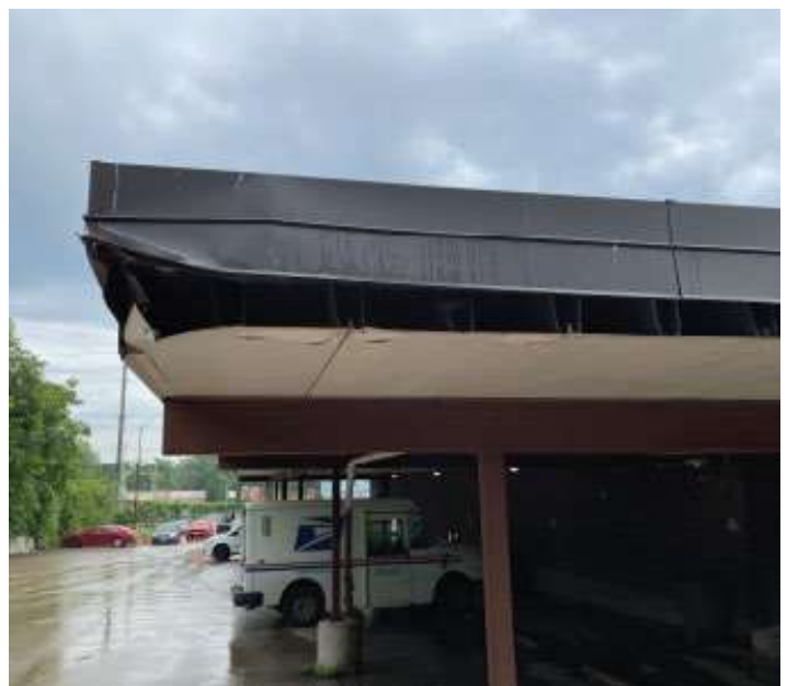
Figure 6. Damaged Awning
